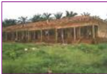
Work in Progress, mid April, 2003.
