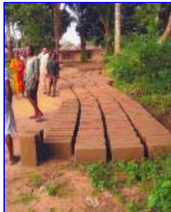
Checking first batch of blocks, November 14th
