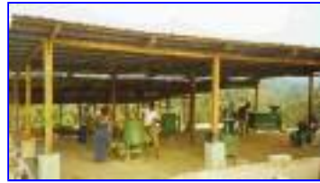
The Working Palm Oil / Cassava Processing Plant
