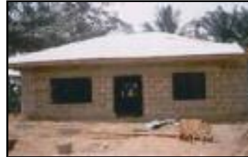
Staff House nearing completion
