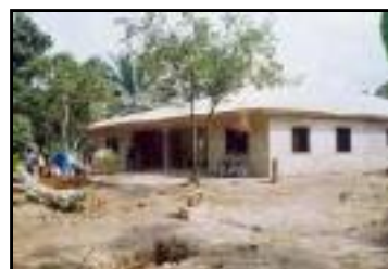
Failed Borehole behind Clinic
