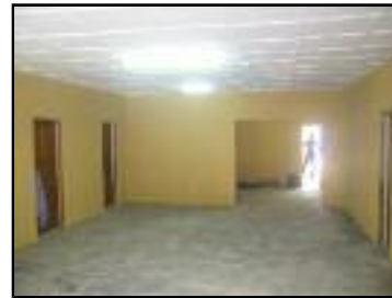
Inside Medical Clinic, still to be equipped
